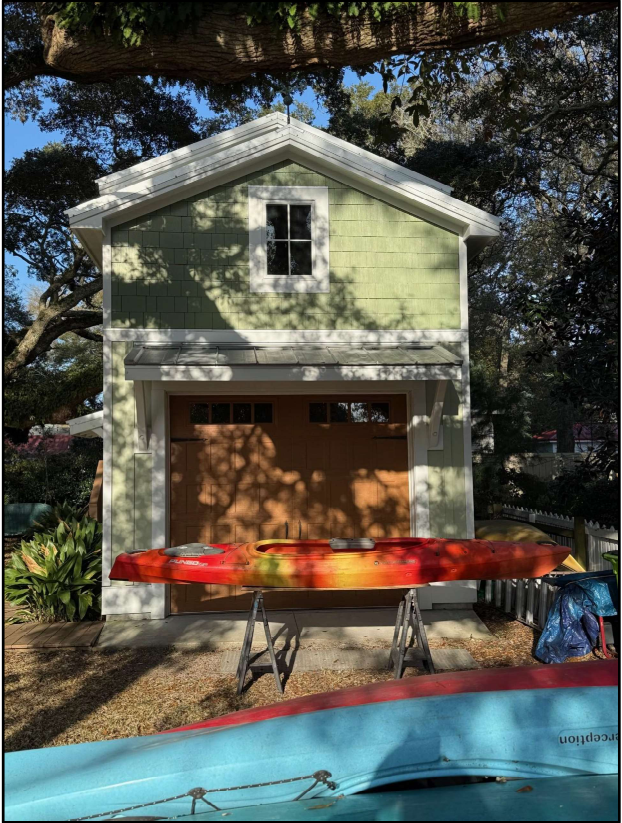
Existing Detached Garage
