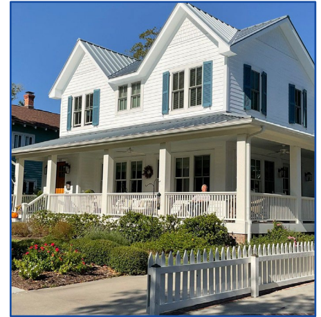
Many of Southport's historic homes have character defining features such as wraparound porches. Craftsmen style porches often include exposed rafters.
