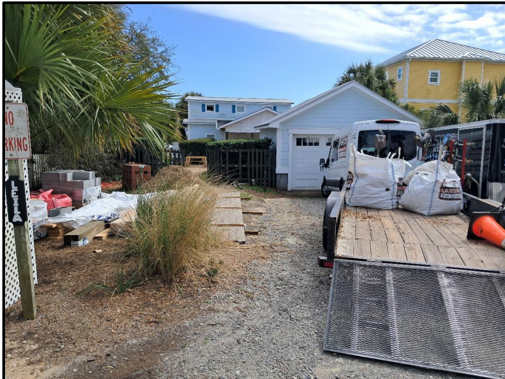
Driveway from Brunswick St
