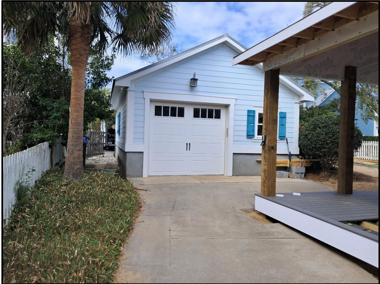
Existing Structure with Garage Door Facing W. Moore St
