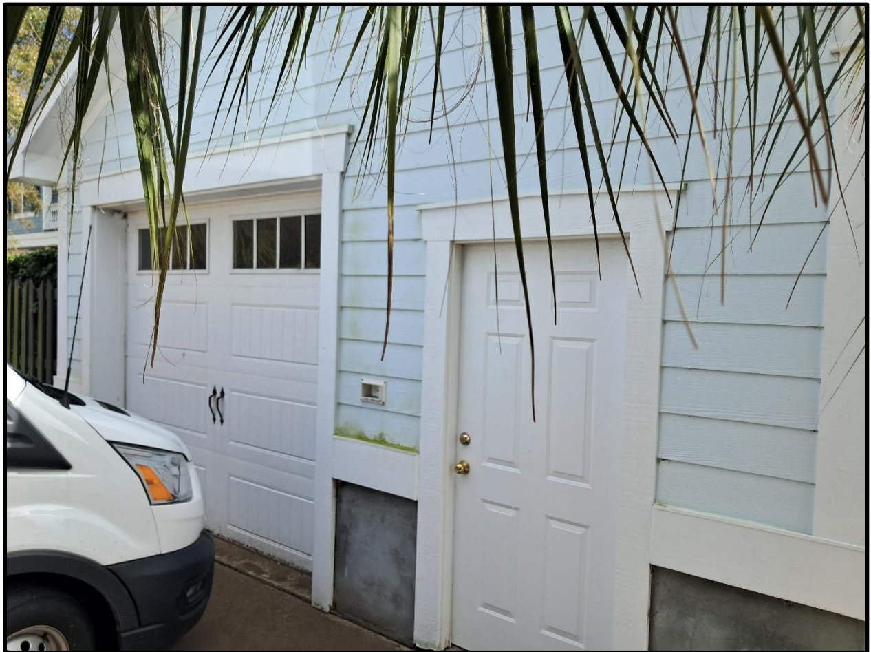
Existing Structure with Garage Door Facing Brunswick St
