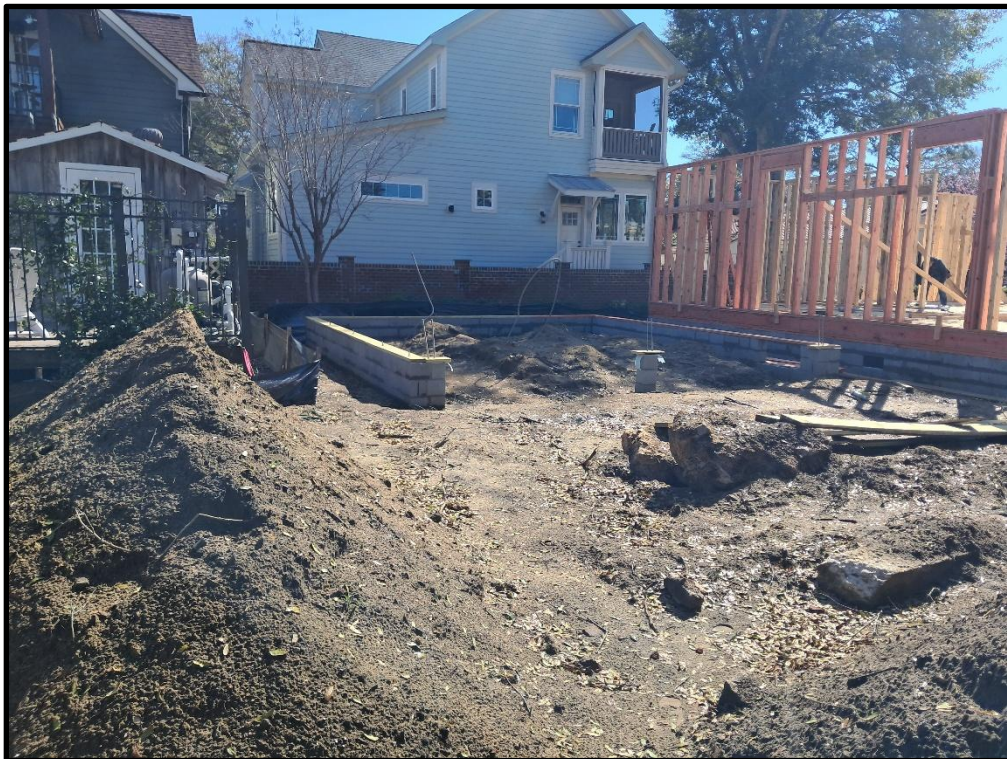
Accessory Structure Under Construction
