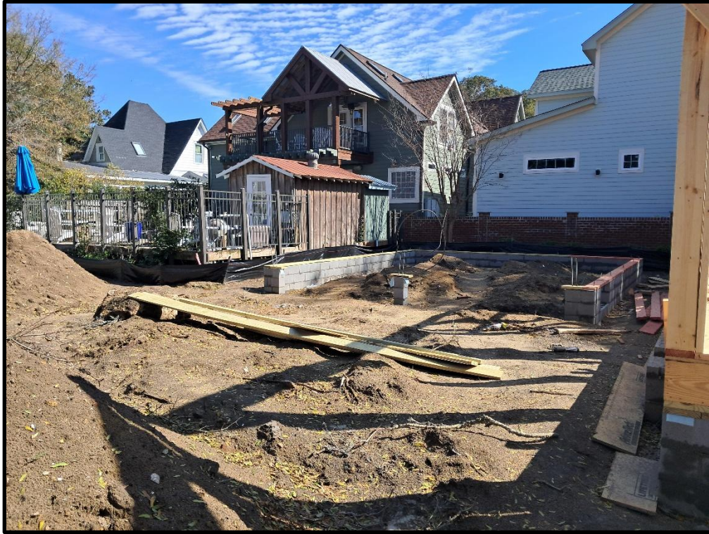
Accessory Structure Under Construction
