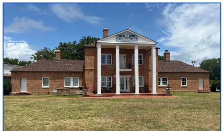
Garrison House (Circa 1804-1809). The only standing structure remaining (in its original location) from Fort Johnston and dates to the Federal period. Image taken on June 18, 2024.
