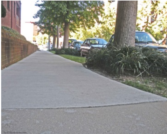
Figure 9: This new smooth and level sidewalk required root cutting within 1.5 times trunk diameter.
