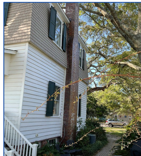
Masonry is a dominant material for chimney construction.
