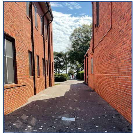
Masonry materials is the dominant building material in the commercial downtown.
