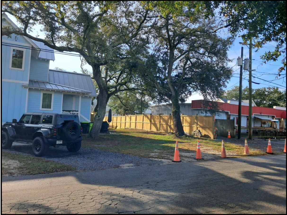
729 N. Atlantic Avenue Street View
