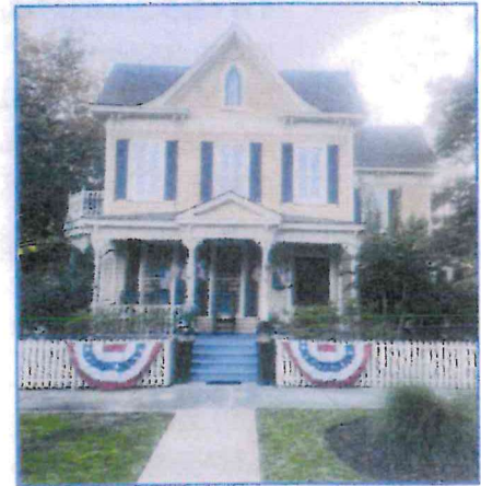
The Adkins-Ruark House has a multi-gabled roof that flares out over deep cornices.
