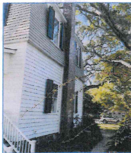
Masonry is a dominant material for chimney construction.
