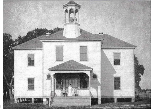
Figure 47: Originally the Brunswick County High School (Circa 1904), this building served as City Hall and is now the Franklin Square Art Gallery.
