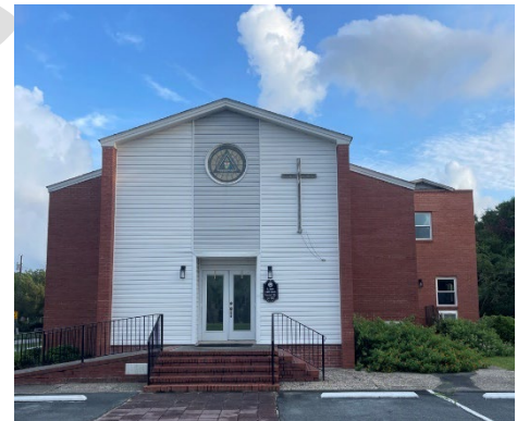
Figure 13: St. James AME Zion Church (Circa 1957, 1961). This is the only African American church listed in the 1867 NC Business Directory and Southport's oldest African American church.
