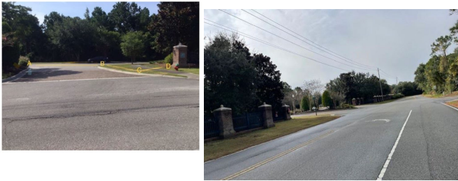
GATE POSITIONING RUARK ENTRANCE View from Ruark, center island at left
