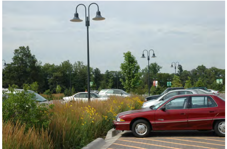
Example of a bioretention area.
