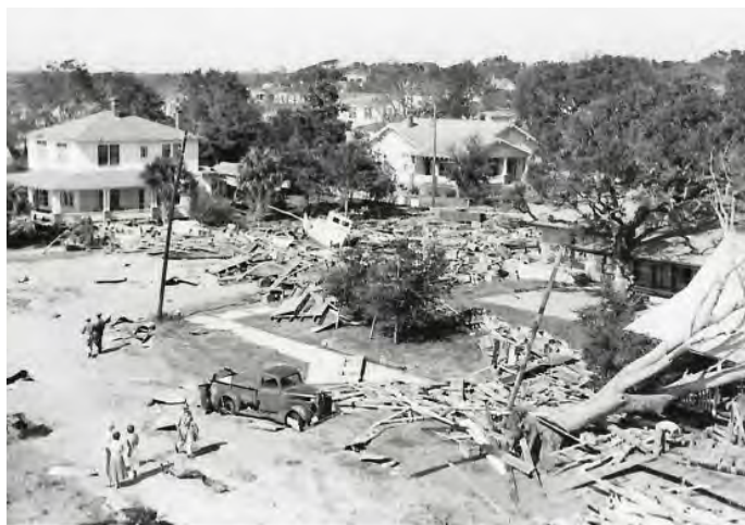
Damage after Hurricane Hazel
