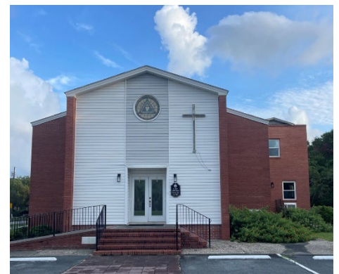
Figure 8: St. James AME Zion Church (Circa 1957, 1961). This is the only African American church listed in the 1867 NC Business Directory and Southport's oldest African American church.
