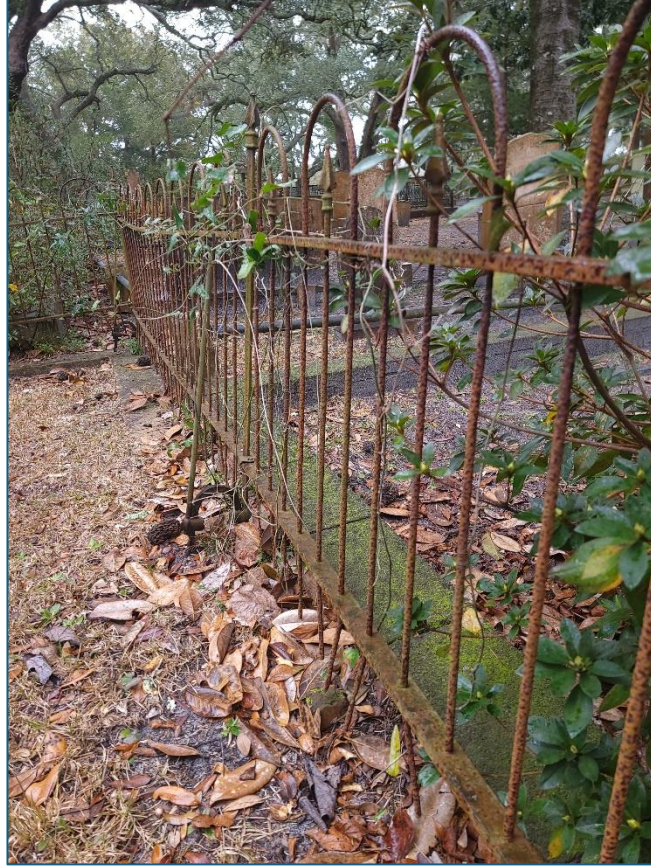
One of the Few Remaining Fences in the Burying Ground
