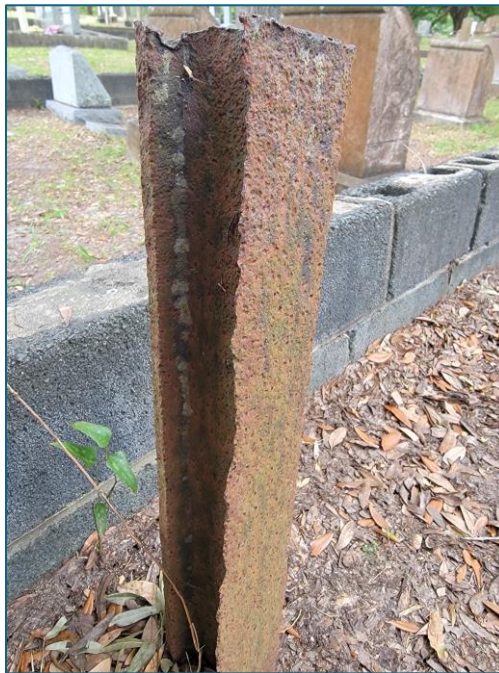
Corroded Railroad Track
