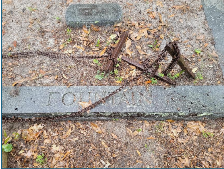
Broken Fence Posts & Loose Chain
