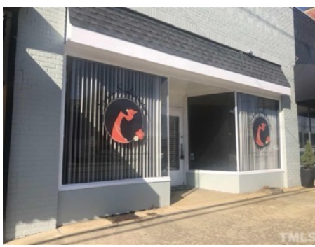
Storefront in Harnett County
